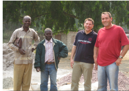
Construction site of a school building in the village, with HSS representative Goetz Heinicke and EU project manager Franck Bisiaux
